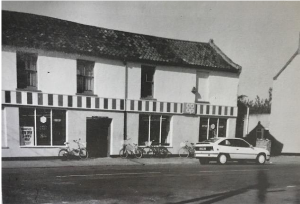
The shopfront in 1989. Christian Enterprise Foundation
