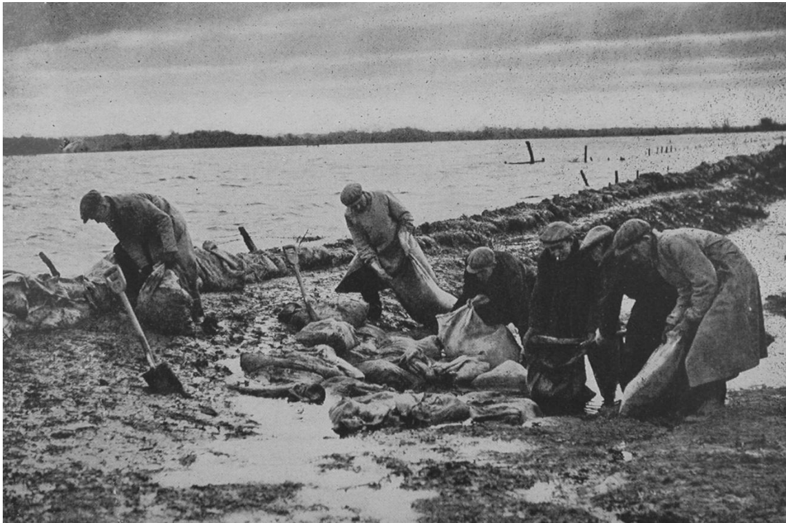
'Repairing the Broken Banks of The River Lode at Lakenheath 1930's' Labourers on Lakenheath Fen. Imagine working under these conditions! LHG Photo Archive.
