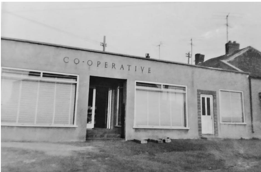
Now the Library, this building housed the Drapery Dept. until it's closure in 1971.
