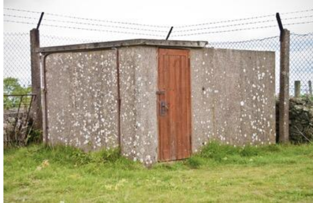
An 'Orlit' Post. A sectional concrete building named after its inventor.
