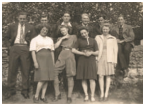
Local men with Land Army girls by the wall of St Mary's church
