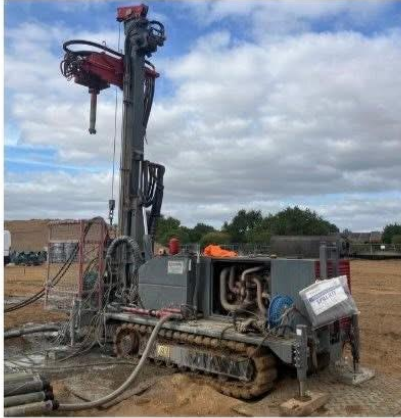
Above: (Left) Boreholes being drilled for the Ground Source Heat Pump
